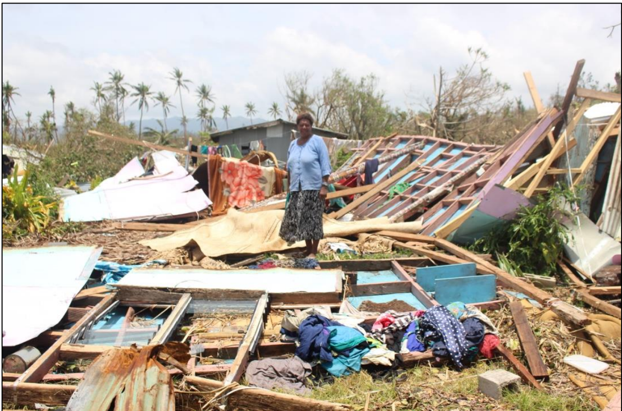
Damage to households on the eastern coast of Viti Levu in Fiji following Cyclone Winston
